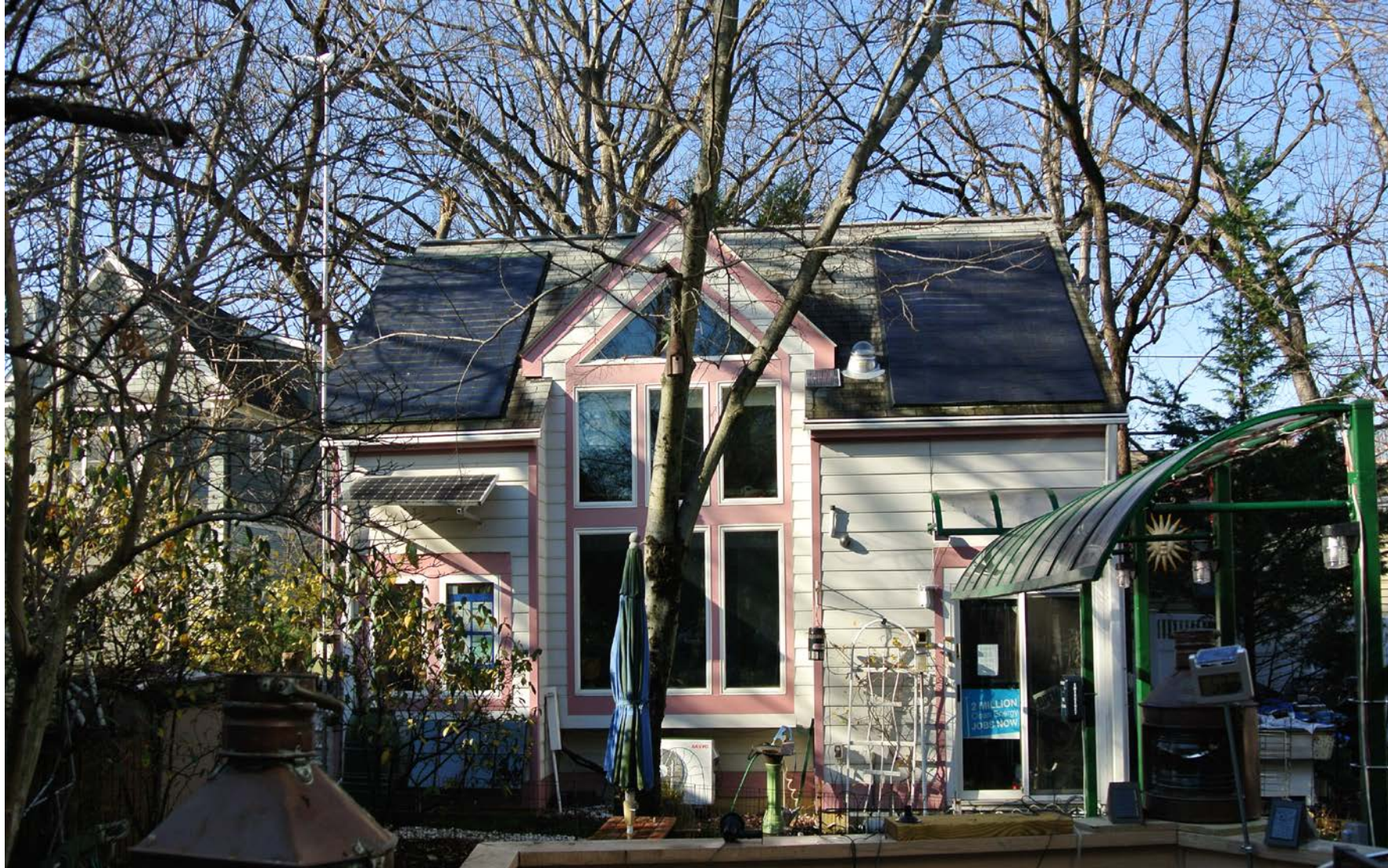
The Stella Group, Ltd. zero energy office (Arlington, VA) UniSolar PV, SW Windpower Turbine, ReliOn Fuel Cell, Gridpoint Battery Bank
