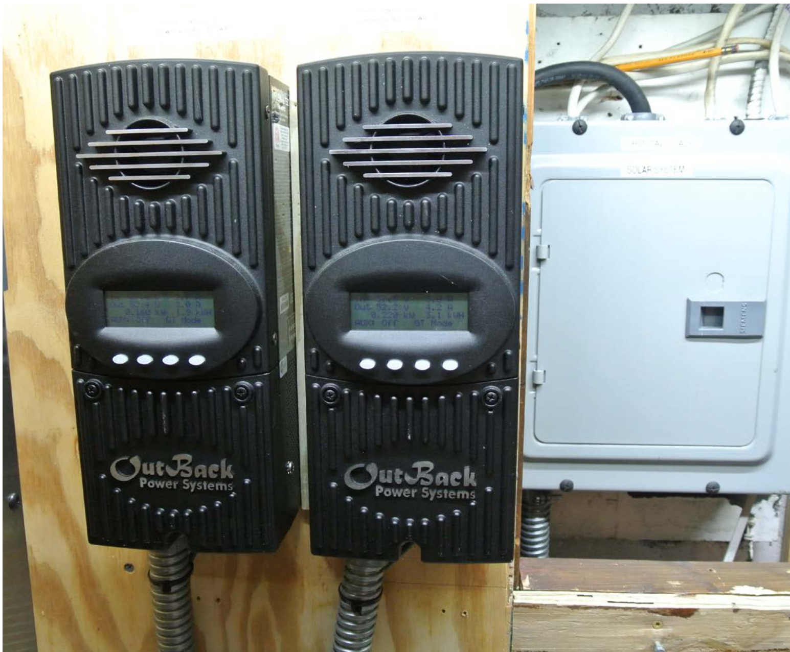
SKLAR HOUSE: OUTBACK CHARGE CONTROLLERS: HIGH & LOW VOLTAGE MODULES
